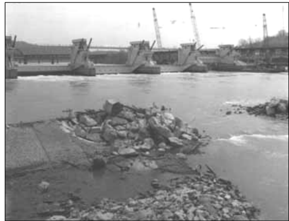
New Braddock Dam with breached old Dam 2 in foreground.
