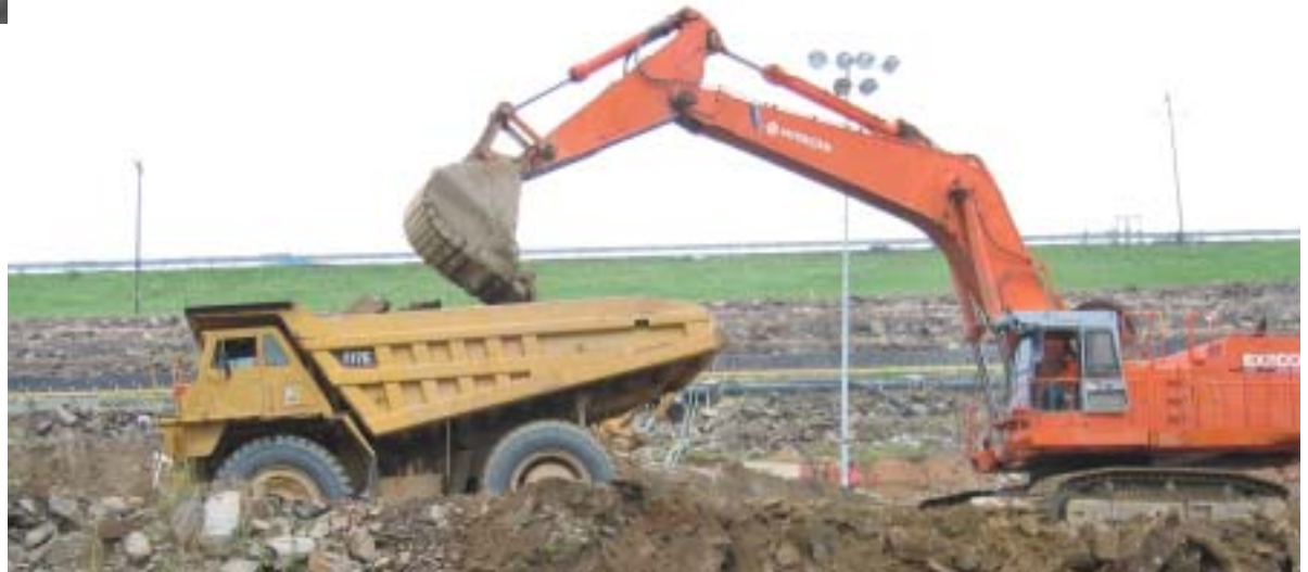
FIGURE 6 Equipment used for construction
