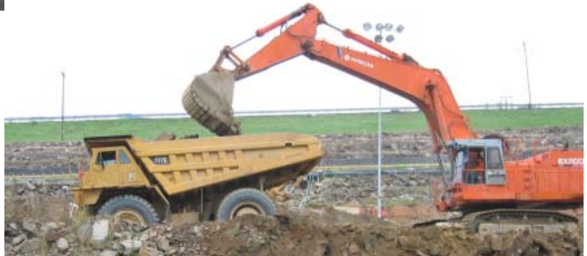
FIGURE 6 Equipment used for construction
