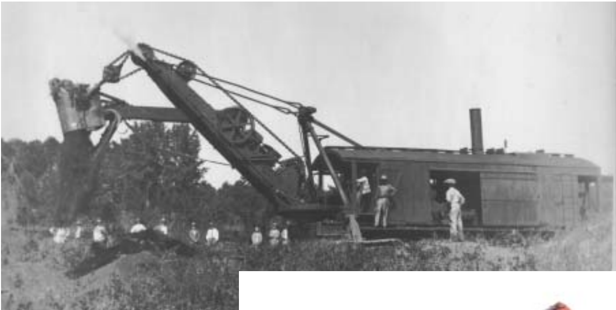
Saluda Dam Construction, 1929
