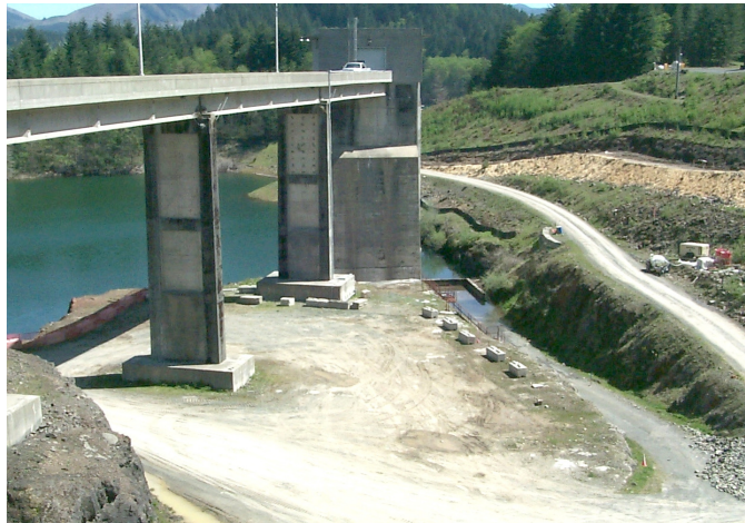
Photograph 2 Excavation Area ( Shannon & Wilson, 2004 )
