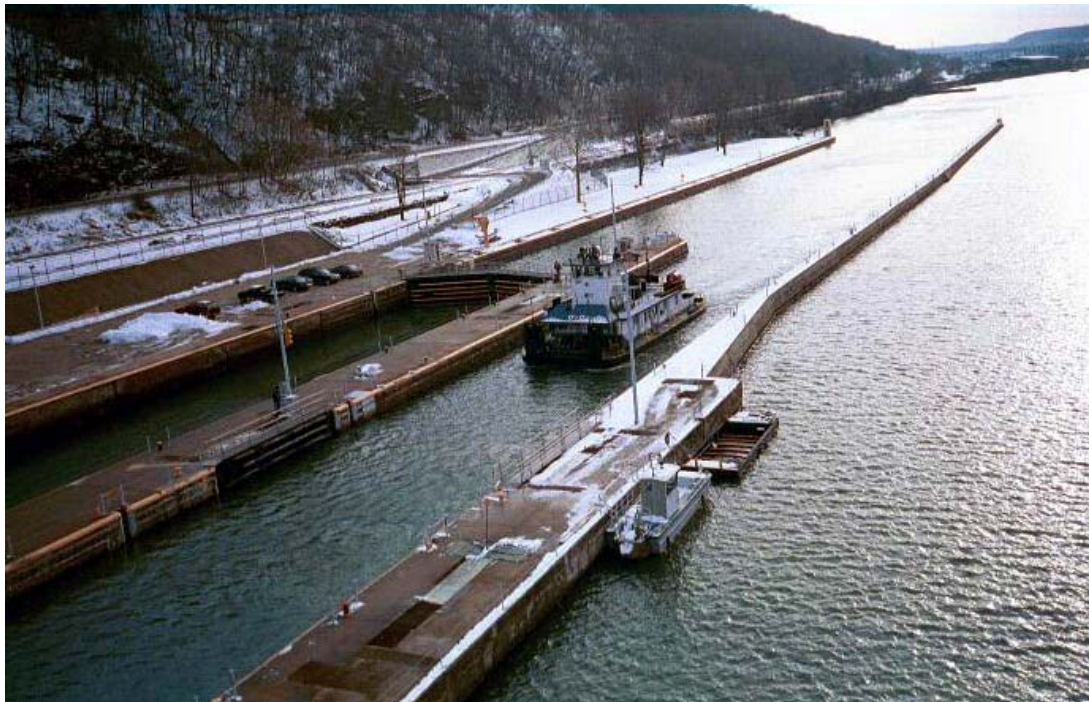
Figure 1. Photo of existing Lock 4 on the Monongahela River, near Charleroi, Pennsylvania
